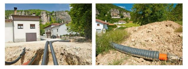
Figure 52. Civil engineering carried out to develop the district network in Sabando.
