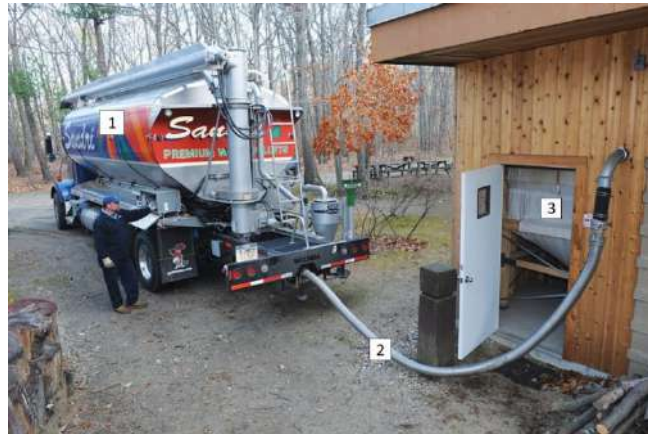
Figure 8. Pellets delivery process with the use of a tanker [14]: 1 – tanker, 2 – delivery pipe, 3 – prefabricated silos.
