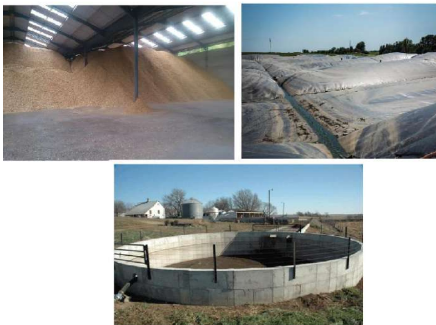
Figure 2: Biomass storage options for different types of biomass: Solid crop waste (top left), sludge (top right) and liquid live stock (bottom)
