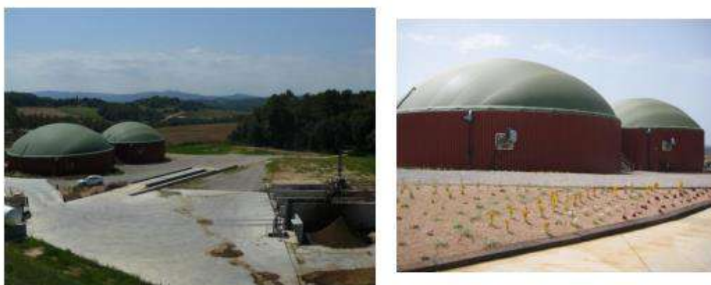
Figure 24. General view of Apergas biogas plant (left), anaerobic digesters (right).
