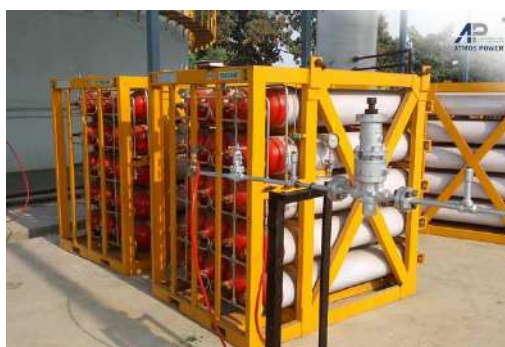
Figure 5: High pressure biogas storage system. Source: AtmosPower Pvt. Ltd. [9]
