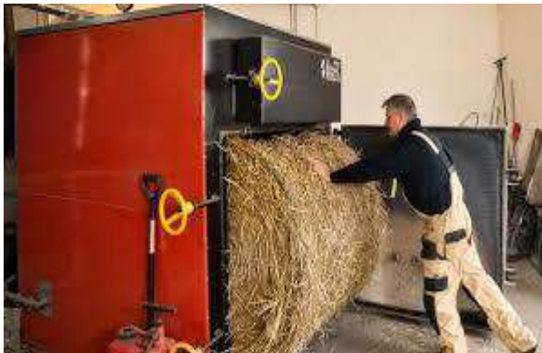
Figure 19. Straw bales/cubes feeding systems [33] [34] : a) manual ; b) automatic.
