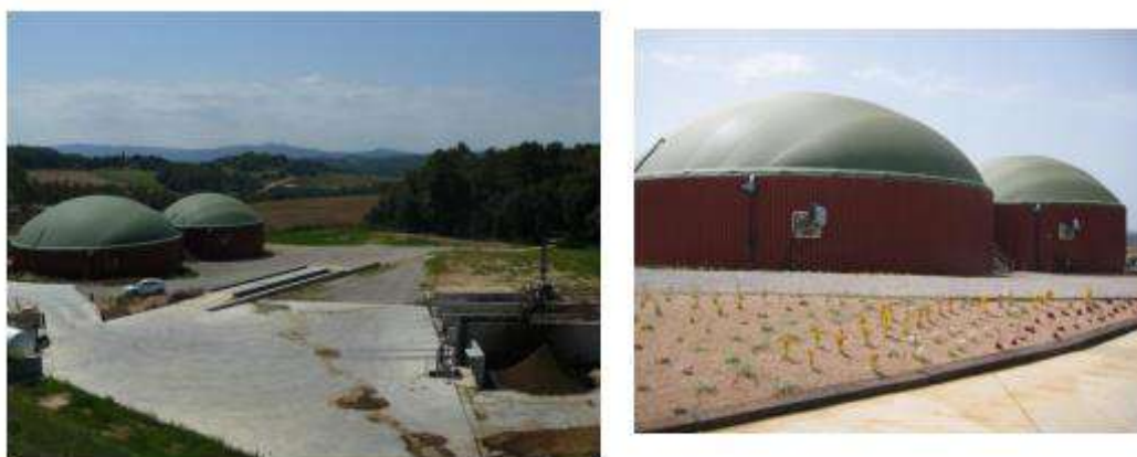
Figure 10: General view of Apergas biogas plant (left), anaerobic digesters (right)
