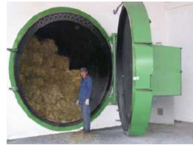
c) biomass boiler
