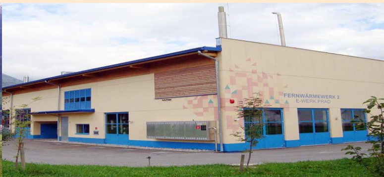
Figure 34. EWP District heating Plant
