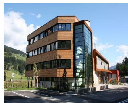
Figure 22. The district heating plant in Toblach (down). The show corridor (up).
