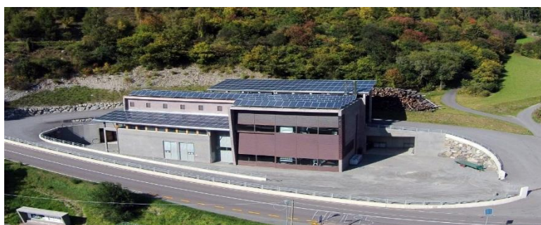
Figure 35. Biomass district heating plant in Taufers in Münstertal
