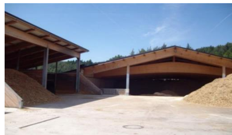
Figure 27. Biomass wood chips storage facility
